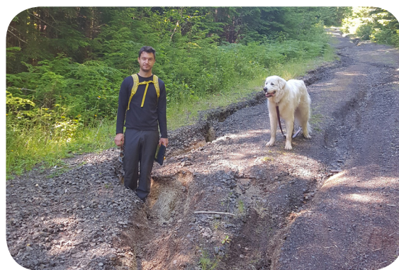
Severe erosion found on a citizen science road survey
