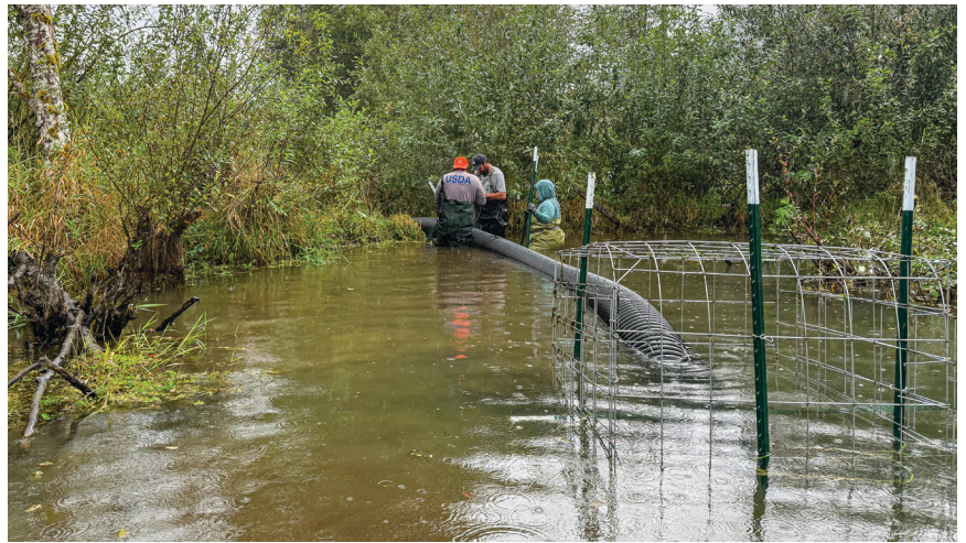
Installation of a pond leveler to prevent flooding of a local PUD's access route. Photo by Cascade Forest Conservancy
